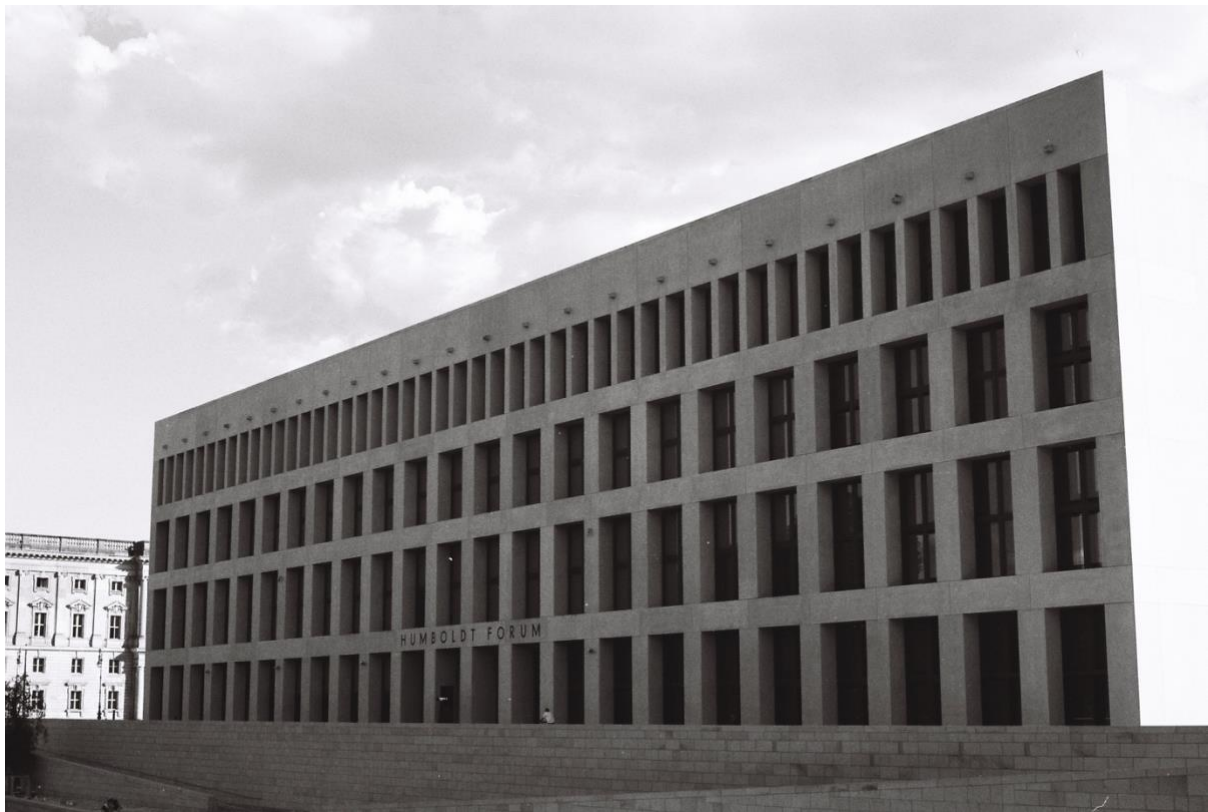
Fig. 6. The contemporary east façade of the Humboldt Forum from the corner of the Marx-Engels Forum.
